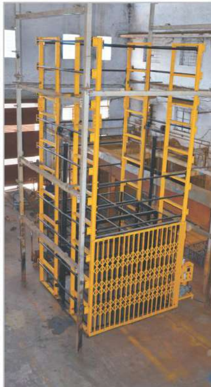
PLATFORM - 2200 X 2200 mm CAPACITY - 2000 Kg. LIFT - 6000 mm
